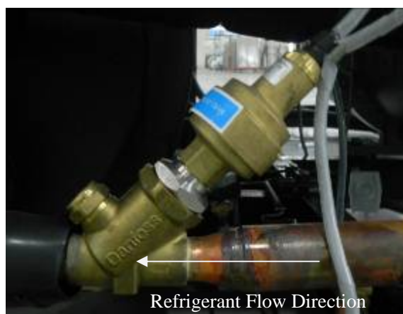
Refrigerant Flow Direction in Electronic Expansion Valve
